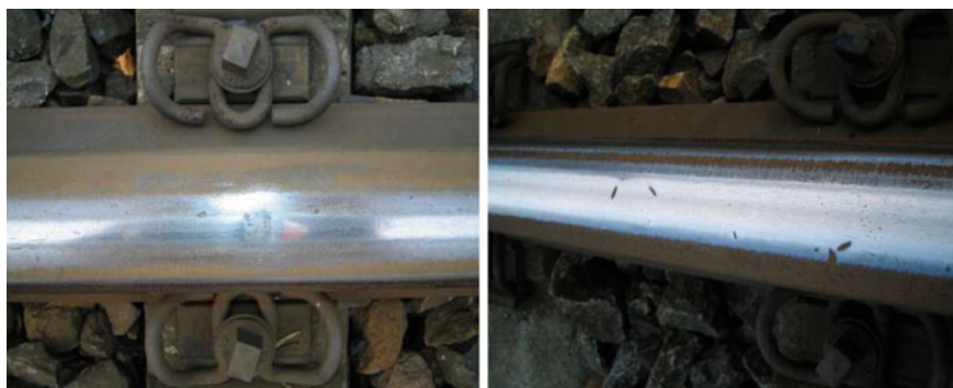
Fig. 26 Local rail surface defects
